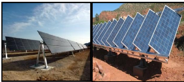
Figure 1. Single-axis and dual-axis solar tracker.
